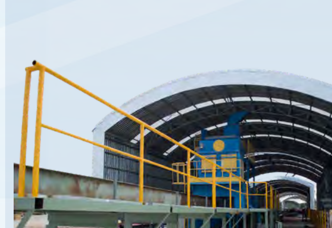
Shot Blasting & Painting Facilities
